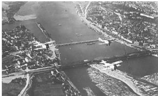
Fig. 2.2. Aerial photography during the activity of Prof. A. Buholcs in Riga (Source: Klētņieks, 2007)
