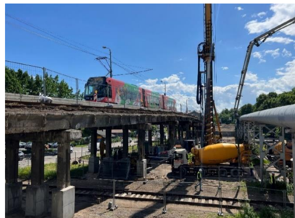
Figure 1. Half of old Brasa overpass, and pail drilling for new construction.
