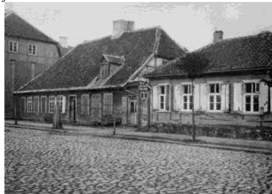
Figure 6. The character of the building construction of Old Jelgava (the end of the 19th century)
