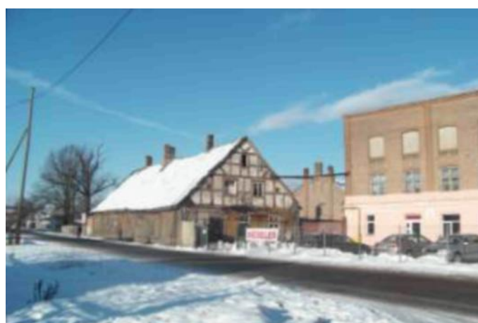
Figure 11. The brick architecture of the old manufacturing buildings adjacent to the wooden building construction on Dobeles street, Jelgava (Author's photo, 2012)
