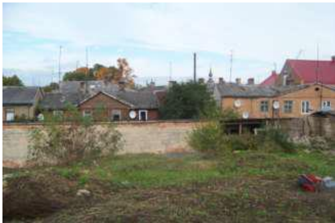
Figure 3. Bauska, Kaleju street. The wooden building construction losing its building, in its place there is a self-growing tree. (Author's photo, 2012)
