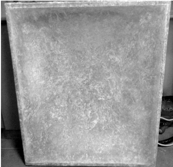
Figure 4. Short glass fiber concrete shell
