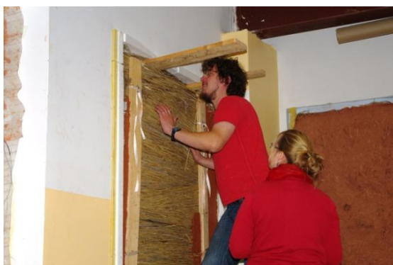
Figure 2. The building of a test wall of horizontal reed (wall S2)
