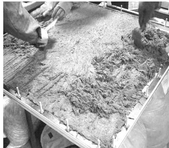
Figure 1. Short glass fiber concrete is evenly placed on the surface of a rubber membrane (pneumatic mould)
