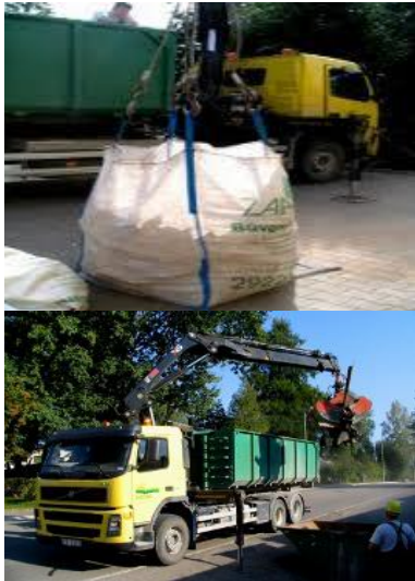
Figure 5. Transportation of construction waste (Collection...)
