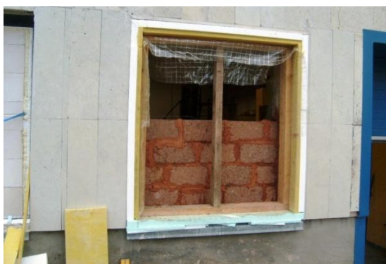
Figure 1. The building of a test wall of light clay blocks (wall S1)
