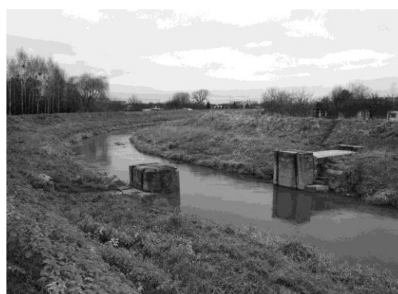
Figure 8. The fortress weir (St. W. X), 2010. (Source: photo by the author, 2010)
