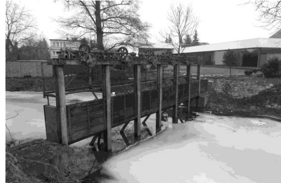
Figure 4. The fortress weir no IV ( Schützenwehr - St. W. IV ) with armour steel plates, 2012 (Source: photo by the author, 2012)
