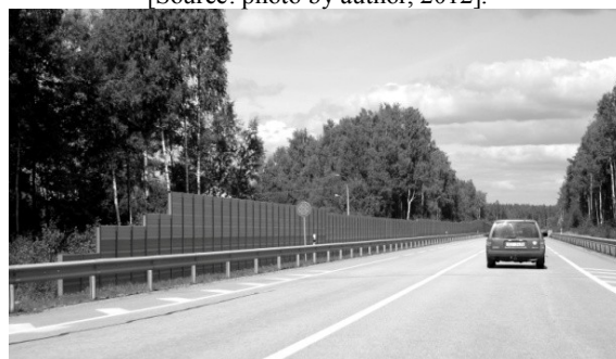
Fig. 9. Sound protection wall, Road Rīga - Salacgrīva [Source: photo by author, 2013].
