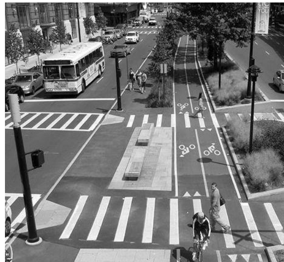
Fig. 4. A bike path with the difference of the carriageway, bike path and sidewalk levels in Copenhagen [Source: photo by author, 2013].
