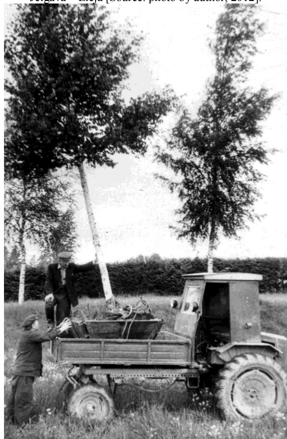
Fig. 3. Tree planting in the road section Pļaviņas – Madona – Gulbene, 1960. Roadside with spruce hedge in background. Foreman Madona CER 10 Kārlis Āboliņš and Osvalds Tauriņš [Source: Latvian road museum].
