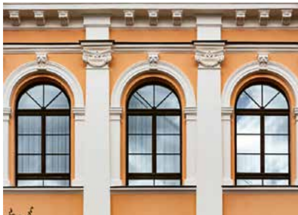
The renovated facade of the Faculty building. The building is an architectural monument of national significance in Zemgale
