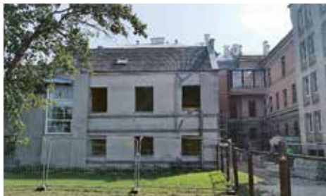
The Faculty building with the small extension before the renovation and the demolition of the extension in April 2022
