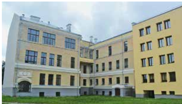
View on the courtyard facade of the Faculty building after the extensive renovation work in 2023
