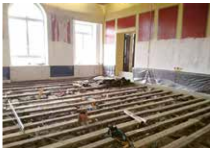
The Faculty hall during renovation in 2017
