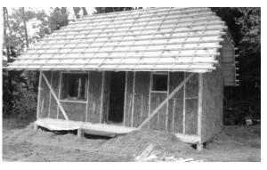
Fig. 4. External appearance of the sauna before rendering
