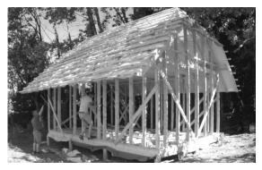
Fig. 3. Timber frame of the sauna is ready
