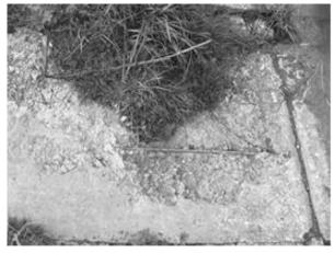
Fig. 1. Pittings and deteriorated concrete covering layer of slabs
