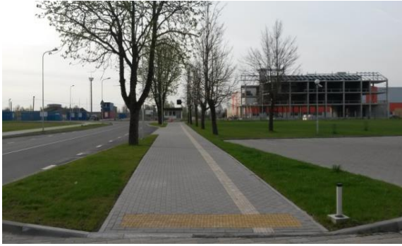
Fig. 1. The old alley of the sugar factory that leads to the new coach factory
